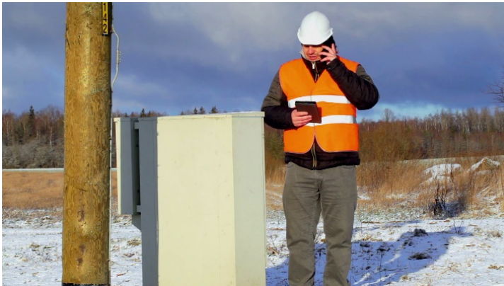
Figure 3a – Servicing Equipment on a Cold Day
